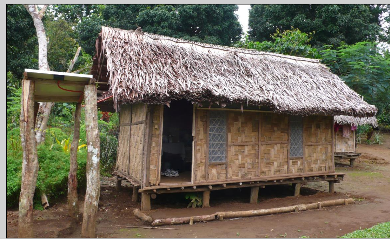
Traditional house with bamboo walling and sago thatch roof, built for project use by members of the Vera'a village community
