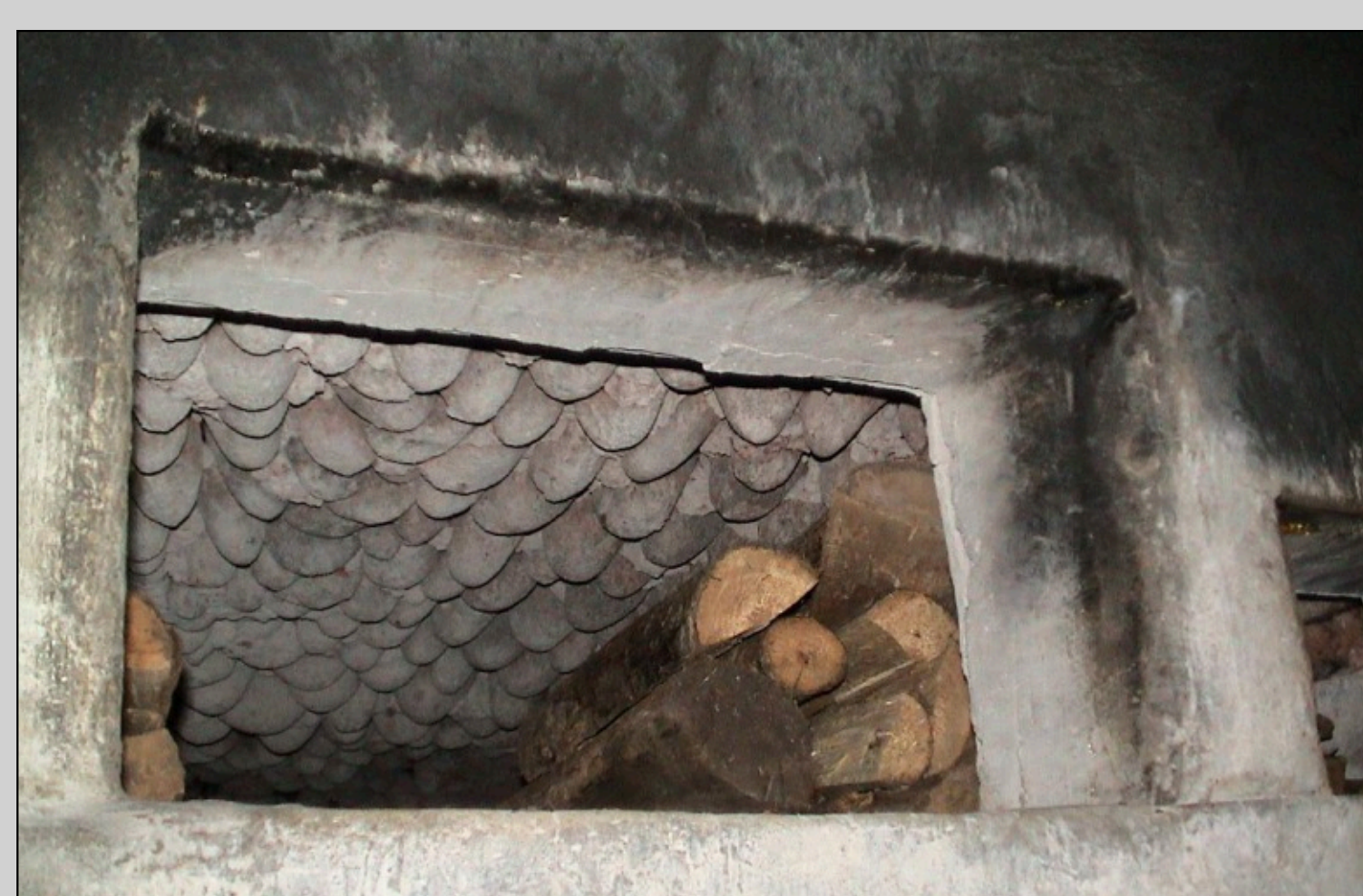
Almost obsolete post-European oven construction with volcanic stones
