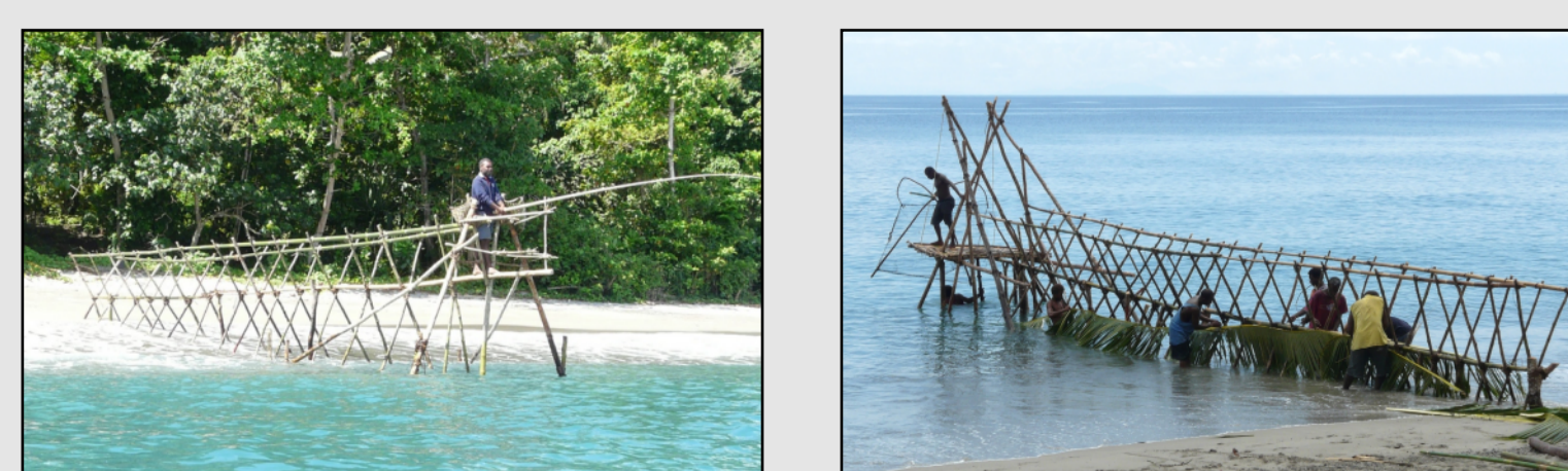
Different designs of fishing bridges are suited for catching different types of fish. Here are two of the fishing bridges built during project workshops: a koku fishing bridge, and a tatata fishing bridge.
